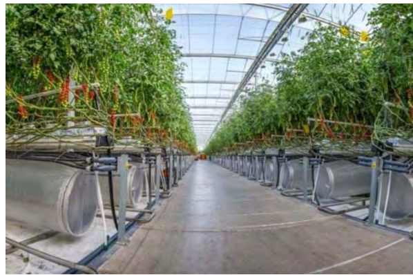
Fig. The SuprimAir greenhouse made by Certhon. Left: the long window that can let air come into the corridor. It includes a wet pad and heating. Right: the sleeves under the gutters.
