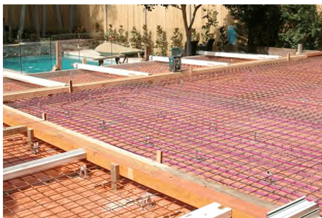
Figure 9: Pictures of in-slab heating
